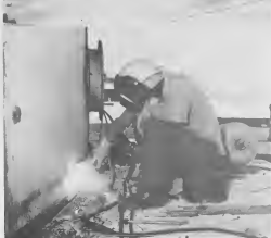
A WORKMAN, above, trims tank plates prior to installation on the bunker station's building site. Applying a weld, left, to one of the storage tank's bottom seams is an employee of Curaçao Dokmaatschappij, one of the bunker station's two contractors. UN TRAHADOR, arriba, ta trim plachinan di tanki promer cu nan worde instala. Aplicando un weld, robes, na bon di un di e tankinan ta un empleado di Curaçoesche Dokmaatschappij, un di e dos contratistanan di e stacion.
